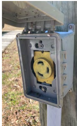
Marine 30-amp outlet without weatherproof gasket and improper cover.
